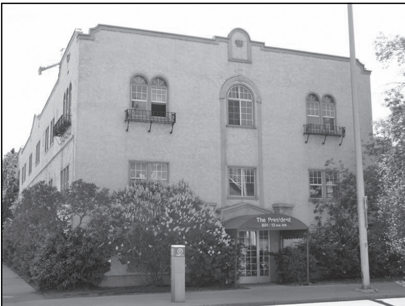
President Apartments, 801 - 12 th Avenue SW.
