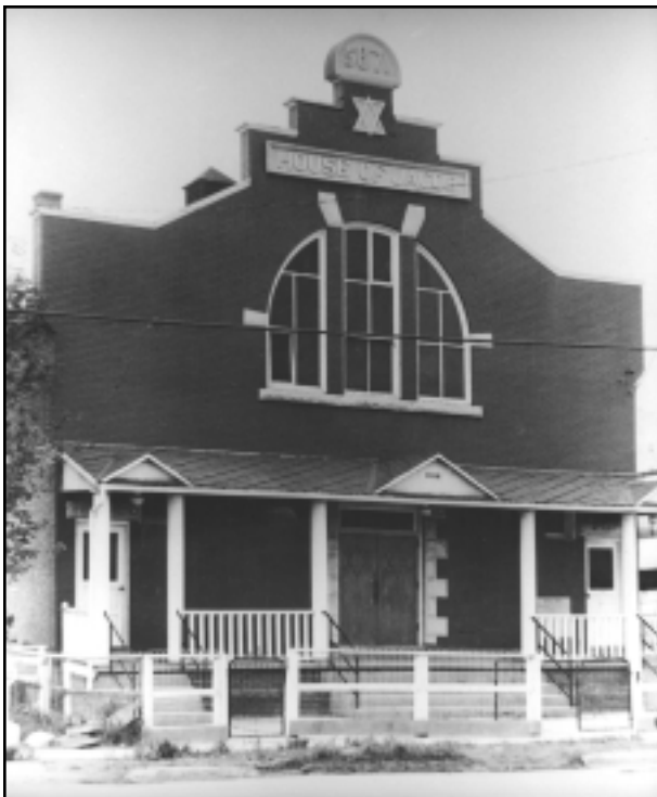
Front of the House of Jacob Synagogue, 1967. The Hebrew date at the pinnacle, 5671, is the equivalent of 1911 in the civil calendar. The 'cornerstone' is visible near the doorway on the far right. Photo: Glenbow Archives, NA-5460-2.
